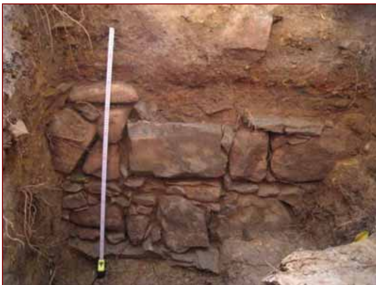
Figure 1: Close up view of the North facing wall in Trench F. The lowest service pipe is visible directly above the wall. 1m scale
