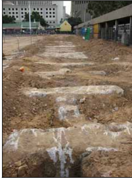
Figure 3: View of the concrete foundations
